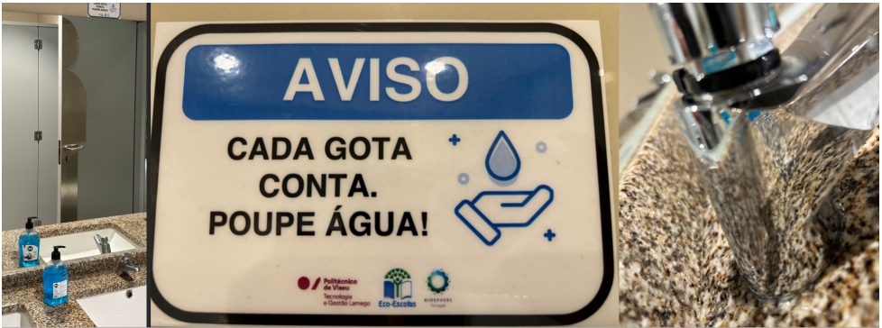
Fig. 17 Signage Placed in Sanitary Facilities and Mechanical Restriction of Water Flow Own elaboration
