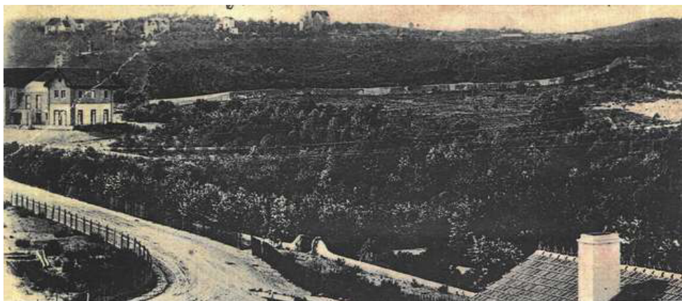
Fig. 2 Quinta do Viana (on the left the Hotel Paris), 1900 Source: Arquivo Municipal de Cascais. PT/CMCSC-AHMCSC/AESP/CJSF/H/EST 056
